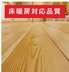
床板：赤松 1階30mm/2階15mm
